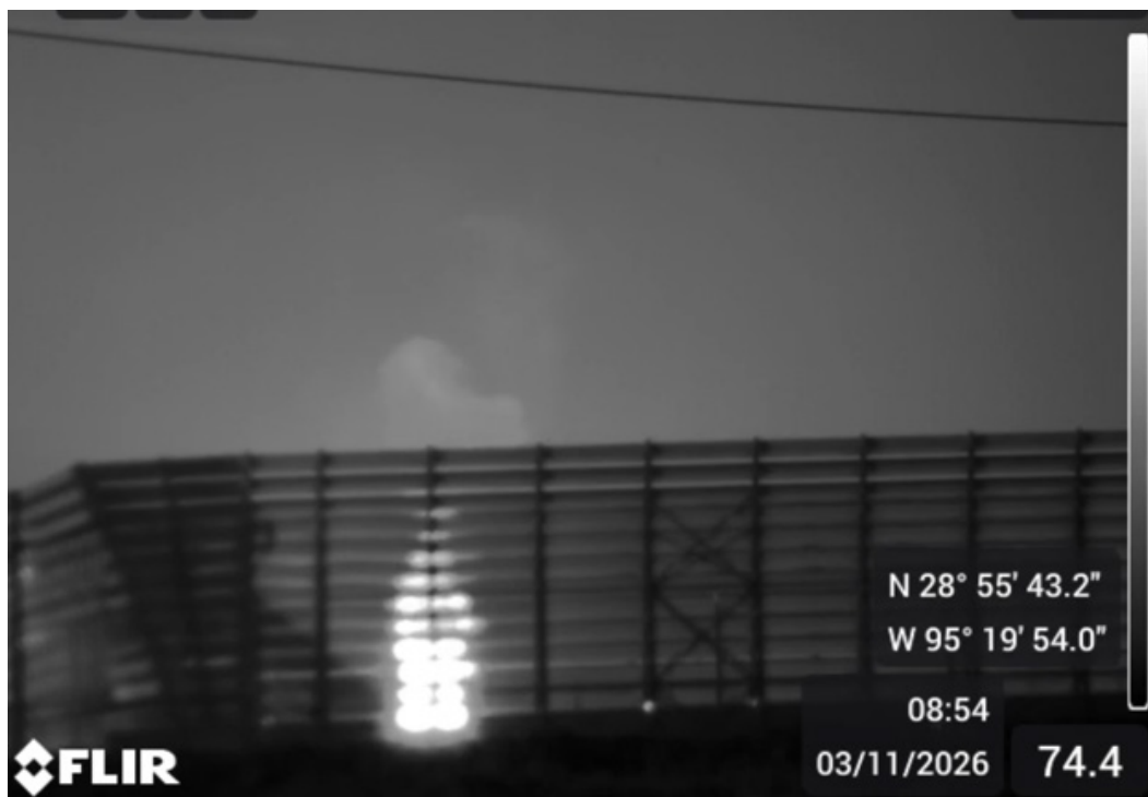
Optical Gas Imaging footage of the Liquefaction flare taken by Sharon Wilson on 3/11/26. The light plume indicates that the flare is not completely combusting gas routed to it. The operation of the flare appears related to the startup at the terminal.
