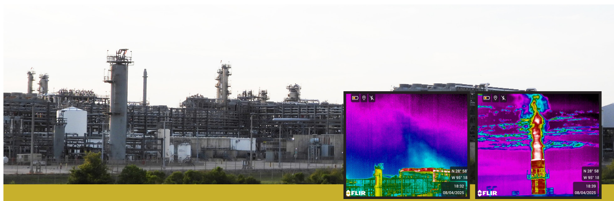
Freeport LNG's pretreatment terminal has multiple sources of emissions documented with optical gas imaging.
